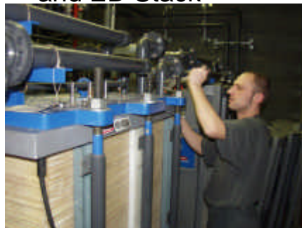
Pump unit of the 20 m 2 plant with sample valve battery at the right side and ED Stack
